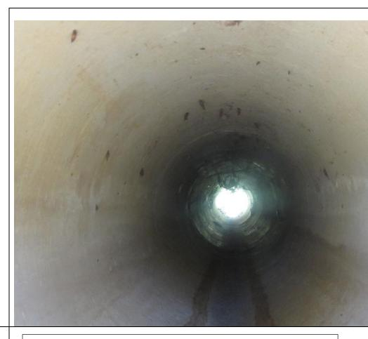
Pipe slightly cracked at outlet.
